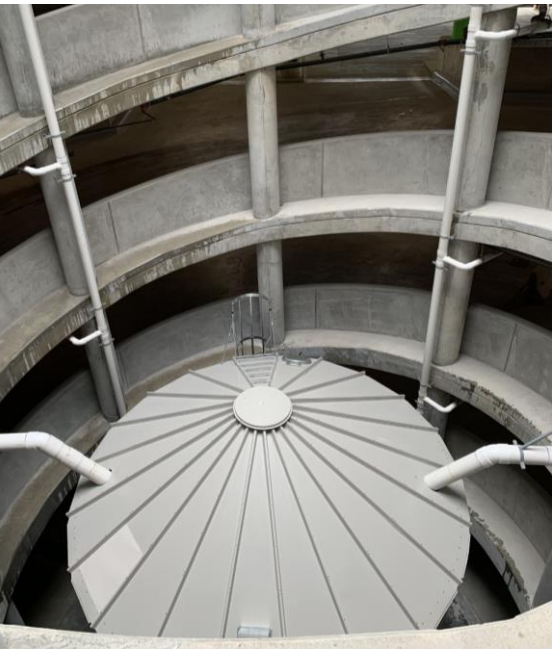
A 50,000-gallon cistern will capture rainwater for landscape irrigation.
