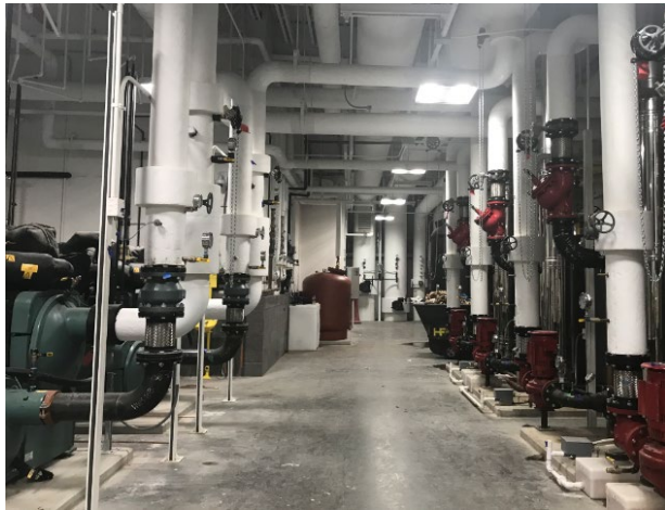
BNA's Central Utility Plant (Courtesy: Fentress Architects)
