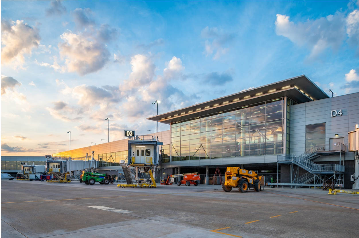
Airside View of Concourse D (Courtesy: Hensel Phelps)
